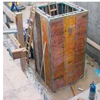
Lift shafts with hot-rolled JORDAHL® anchor channels approved by the Building Approval, can be loaded dynamically, good alignment of the lift guide channel in the shaft.
